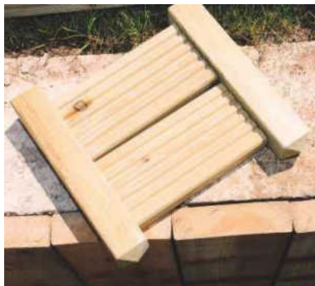
STEP 7. Place the parts together to check everything is correctly sized
